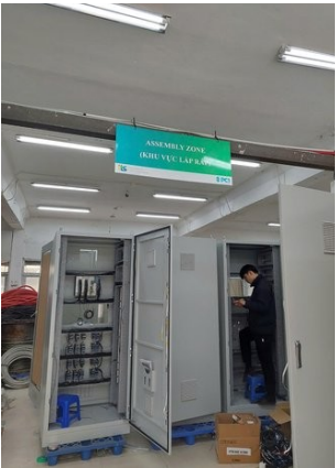
Warehouse and workshop
